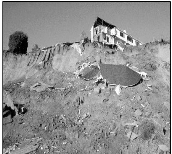
Source: American Planning Association Landslides
