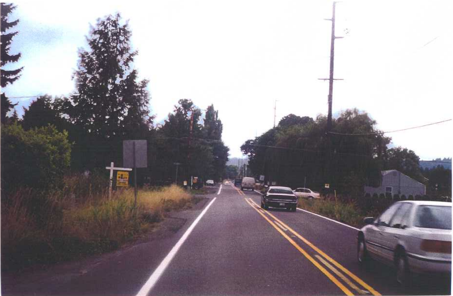
FIGURE A-7 SW 170th Ave. North of SW Farmington Rd. - Existing
