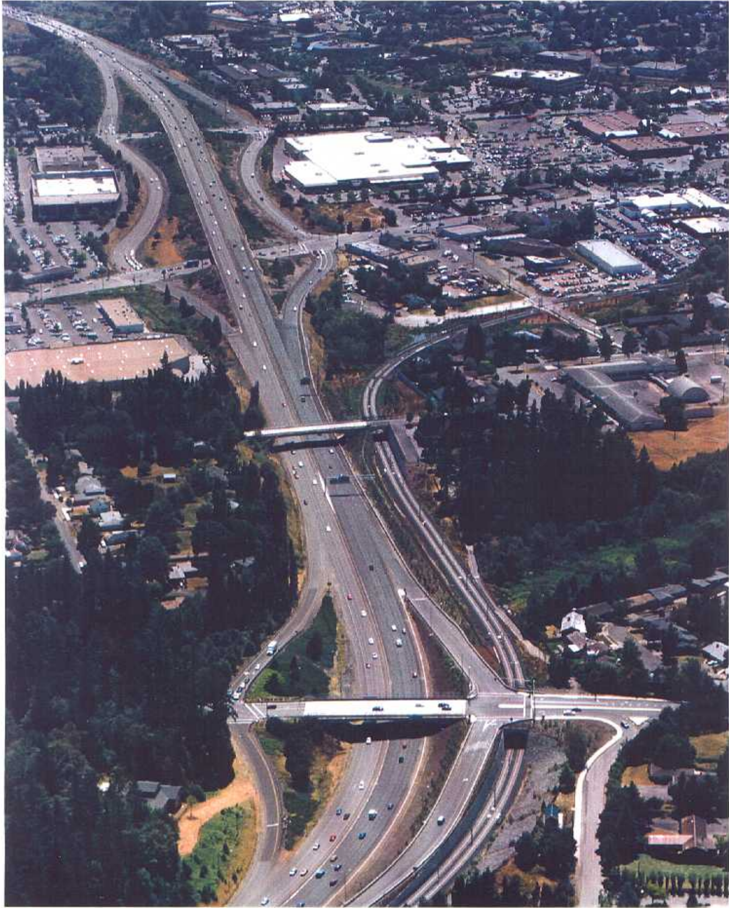
FIGURE A-1 ORE 217 at SW Walker Road - Existing
