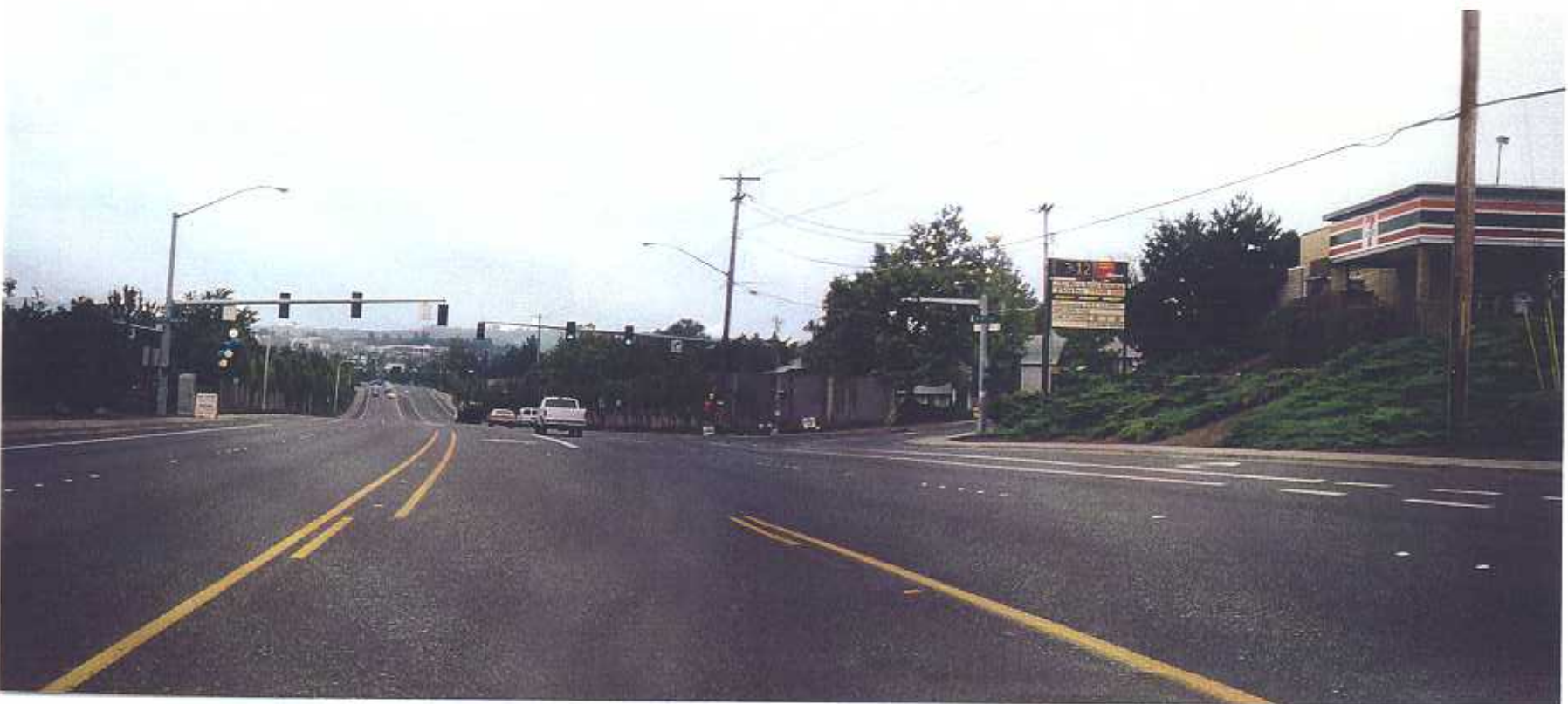
FIGURE A-11 SW Scholls Ferry Rd. East of SW 125th Ave. - Existing
