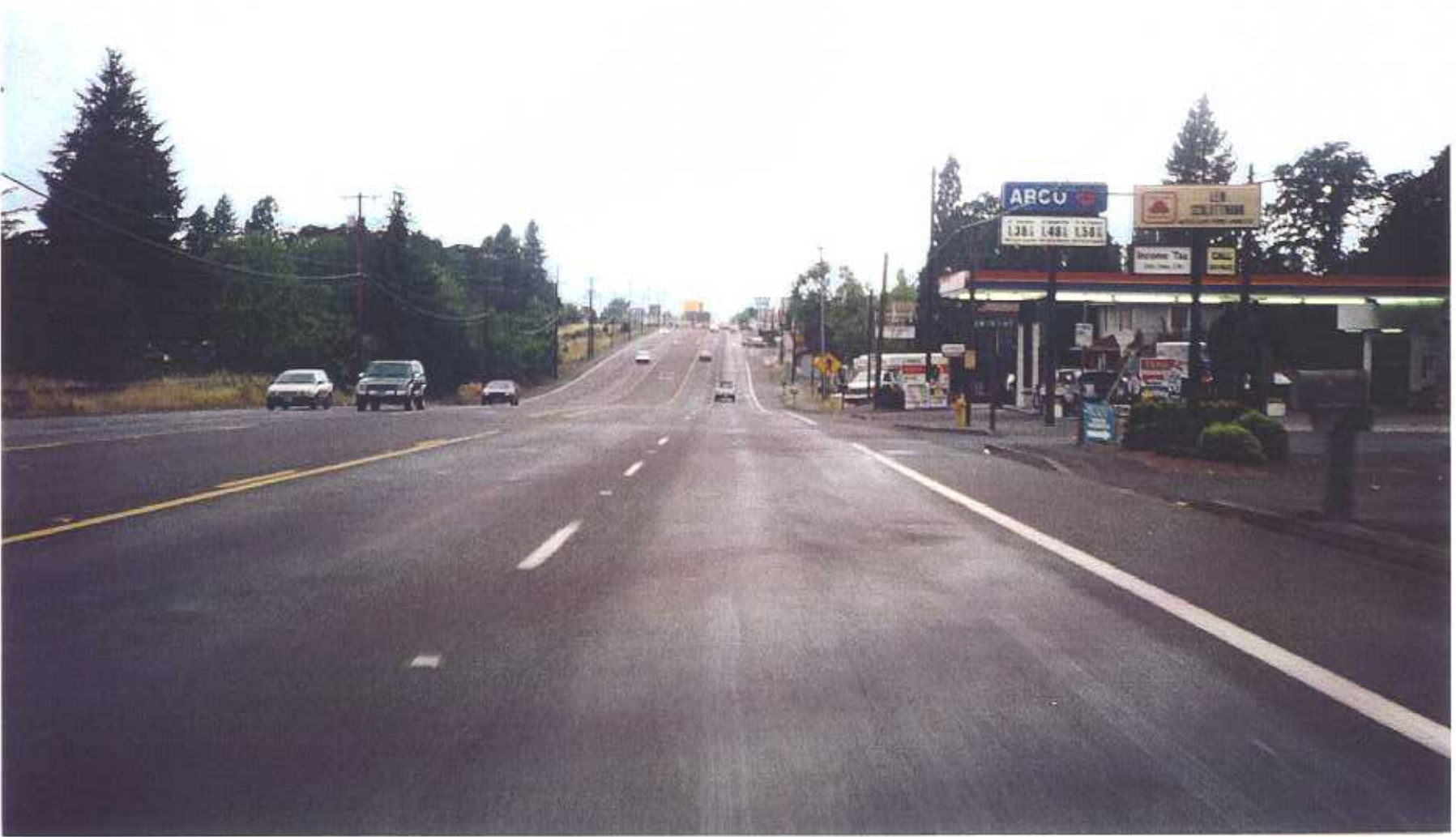
FIGURE A-9 SW TV Hwy. West of SW 170th Ave. - Existing
