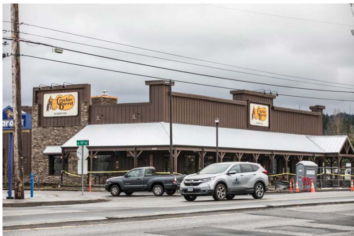
TIMES PHOTO: JONATHAN HOUSE - Cracker Barrel in Beaverton
