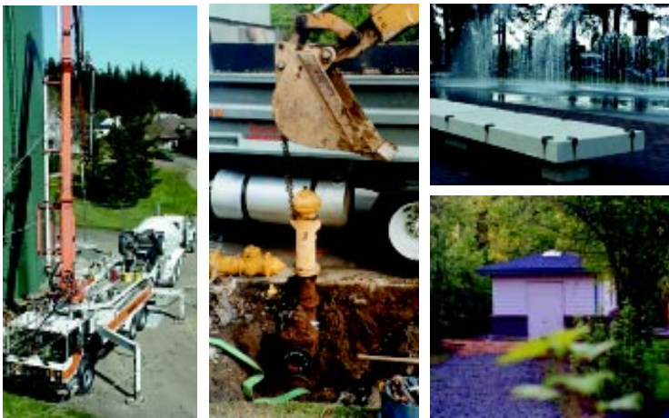
Repair of 5MG tank, hydrant replacement project, Beaverton's new fountain, Murray Hill pump station
