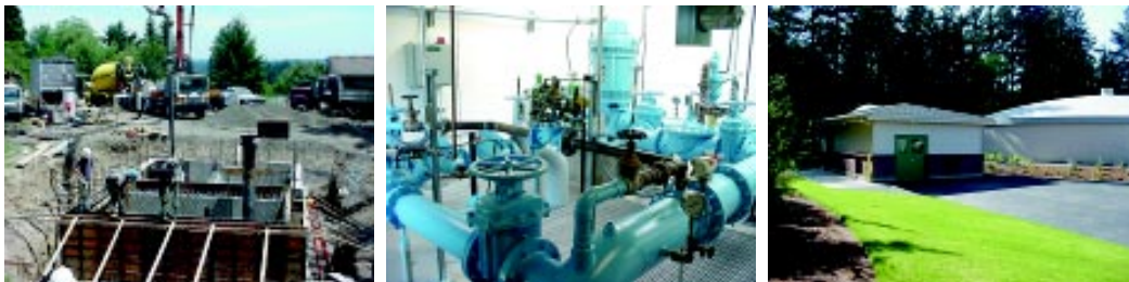
ASR #2 under construction, piping, after initial landscaping
